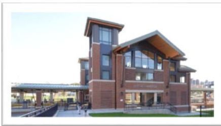
1 Meriden Transit Center
