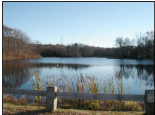
Lower Black Pond – New Dam
