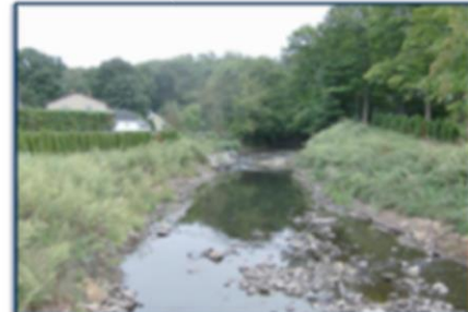
Harbor Brook Channel Improvements
