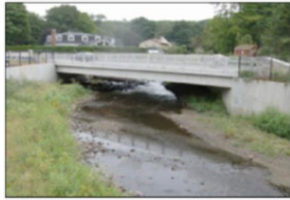
6 Bridge Replacements & 2 Relief Culverts
