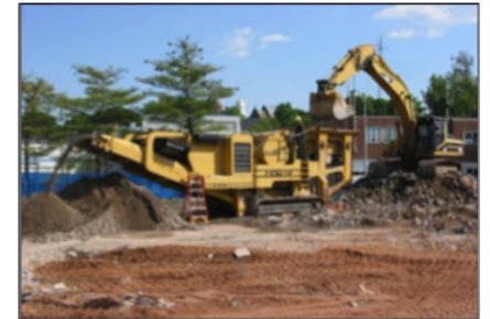
Property Acquisition, Demolition and Flood Proofing
