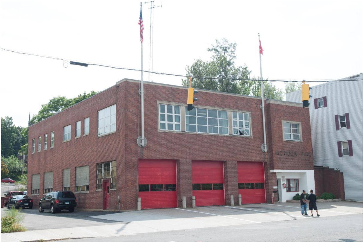
Modern – Meriden Fire Headquarters, 51 Pratt Street
